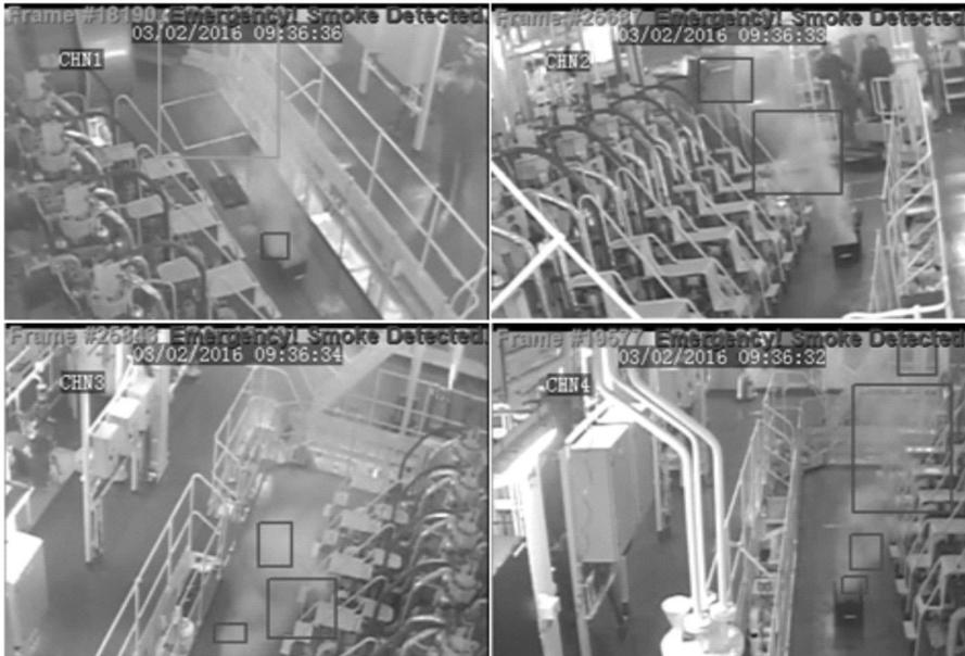
Figure 8: Video smoke detection using 4 different angle cameras in a 3 sec time gap
