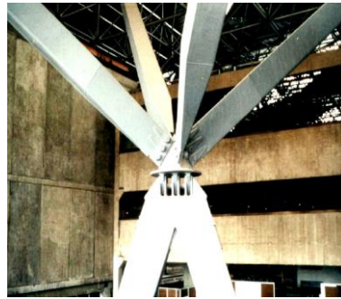
Figure 6 Bolted connections of column branches [3]
