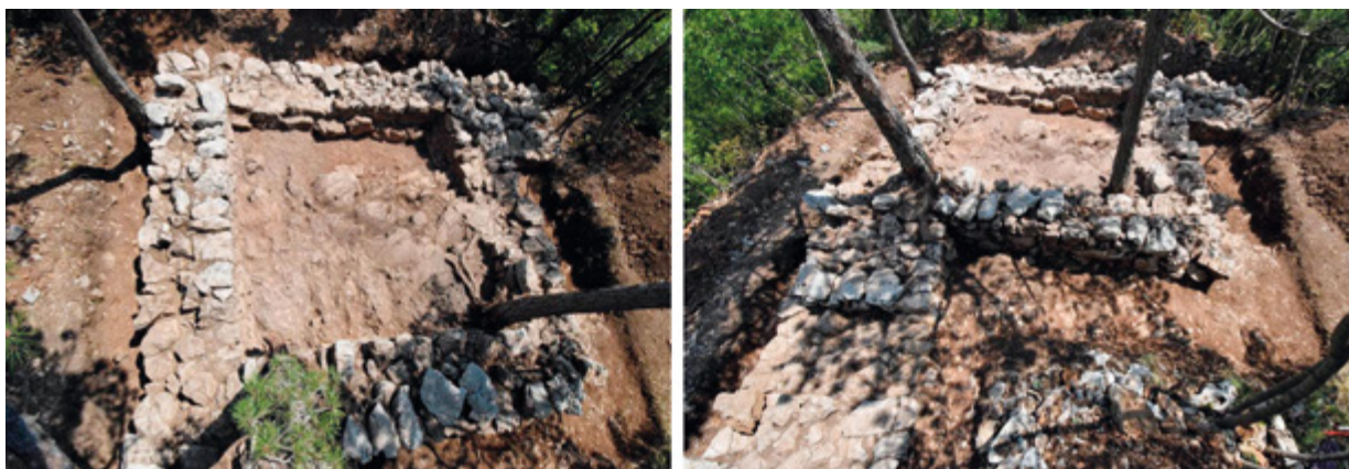
17. Pogled na istražene građevinske strukture na lokalitetu Obrovac - Kalić (snimio T. Percan) View of the investigated buildings at the Obrovac–Kalić site (photo by T. Percan)
