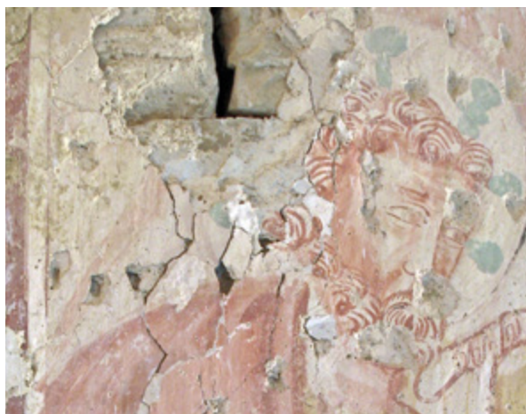
6. Pucanje arriccio i intonaco odvojenih od nosača (snimio B. Hacker, 2009.) The cracking of arriccio and intonaco detached from the support (photo by B. Hacker, 2009)
