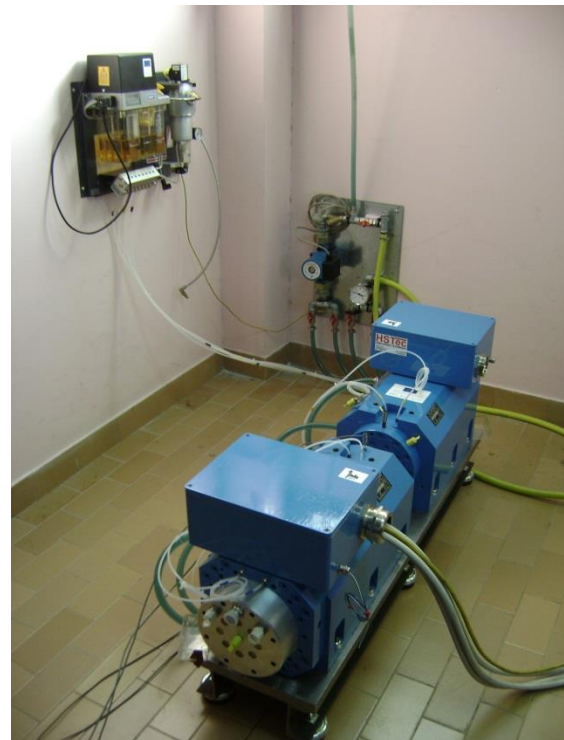
Figure 8. High-speed motor-generator group with a lubricating oil unit and cooling system
