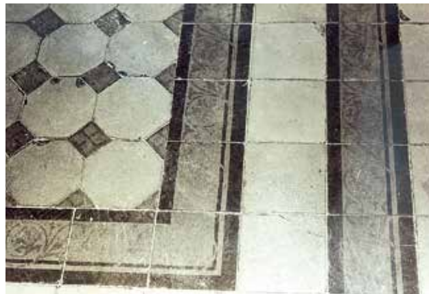
23 Crkva Gospe van grada, detalj poda od keramičkih pločica, stanje 1997. (foto: I. Šprljan) Church of Our Lady Outside the Walls, detail of the floor from ceramic tiles, state in 1997 (photo: I. Šprljan)
