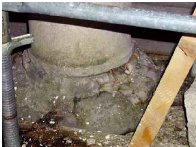
5 Pročelje, prizemlje, baza stupa, stanje prije radova (foto: I. Šprljan) Frontispiece, ground floor, pillar base, condition prior to works (photo: I. Šprljan)
