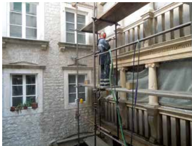
22 Čišćenje kamena metodom retuš-pjeskarenja pomoću staklenog pudera (foto: Š. Glavan) Stone cleaning by retouch-blasting method using glass powder (photo: Š. Glavan)
