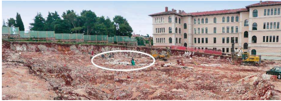
Figure 3. Mine field in construction pit, research location Rovinj
