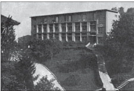
FIG. 9 NEUMANN, ZLATKO: TBC PAVILION, "DR MLADEN STOJANOVIC HOSPITAL", TODAY "SESTRE MILOSRDNICE" HOSPITAL, 29 VINOGRADSKA ST, ZG, HR, 1954, CONTEMPORARY PHOTOGRAPH
