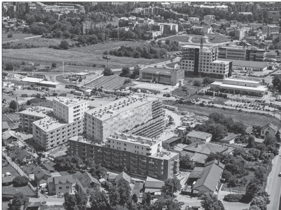
SL. 8. PROGRAM DRUSTVENO POTICANOG NAJMA STANOVA [PON]: STAMBENE ZGRADE, KLARA, ZAGREB FIG. 8 STATE-SUBSIDIZED HOUSING PROGRAM FOR RENT [PON]: APARTMENT BUILDINGS, KLARA, ZAGREB
