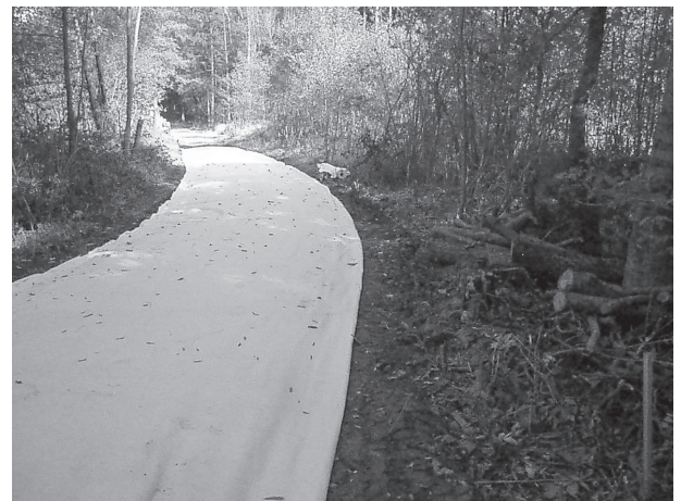
Fig. 5 The layer of brown chips enclosed in geotextile
