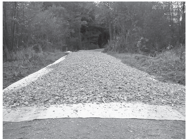
Fig. 4 Brown chips laid on geotextile and sloped and compacted subgrade
