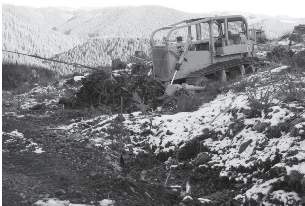
Fig. 1 Bulldozer using a mobile anchor
