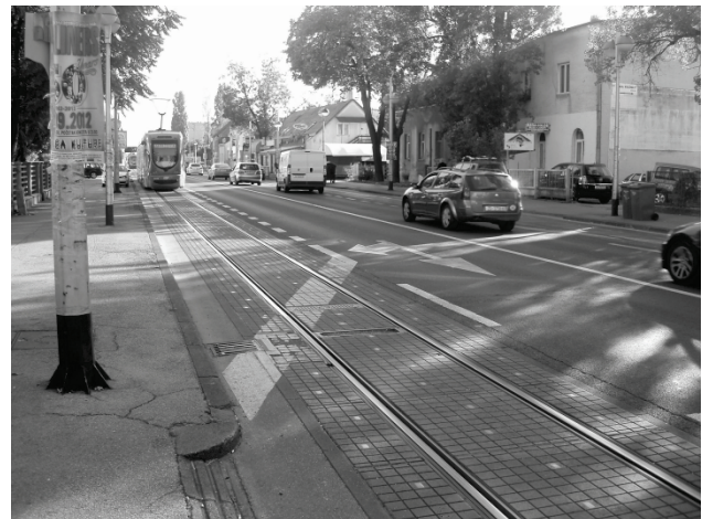
Figure 1 An example of tram lanes integrated into road network – transition from yellow lane (farther) to white lane (closer)
