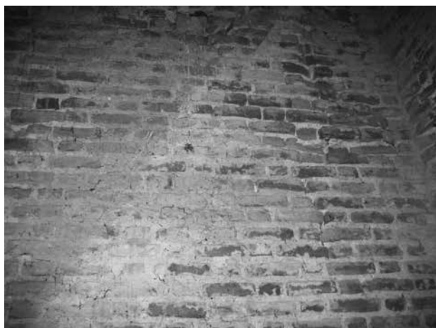
7. Kloštar Ivanić, crkva sv. Marije, zvonik, treći kat, sjeveroistočni kut, razlike u zidu (foto: M. Cepetić Rogić) / Kloštar Ivanić, church of St Mary, belfry, third floor, northeast corner, differences in brickwork (photo: M. Cepetić Rogić)
