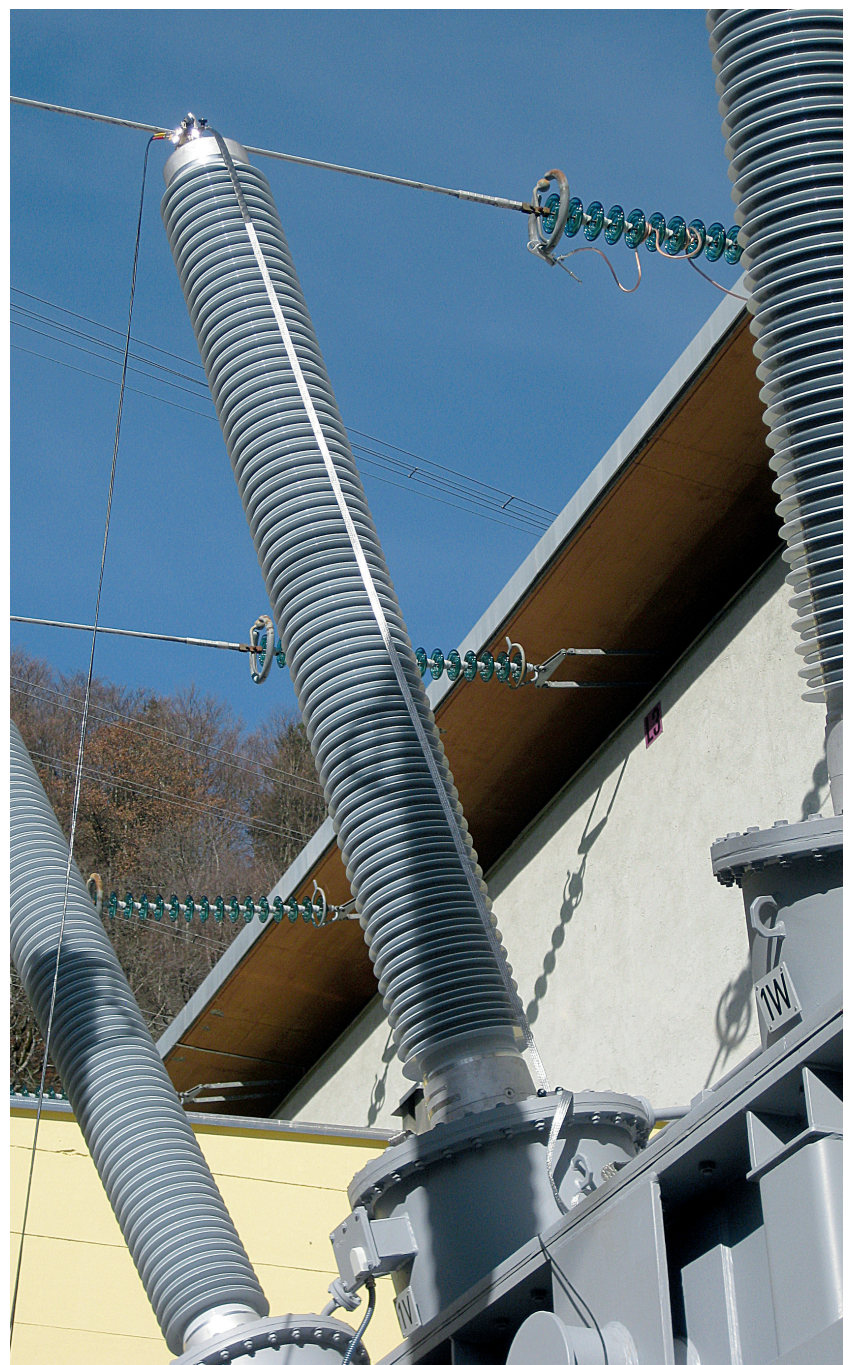
Figure 7. Example of shortest braid connection concept
