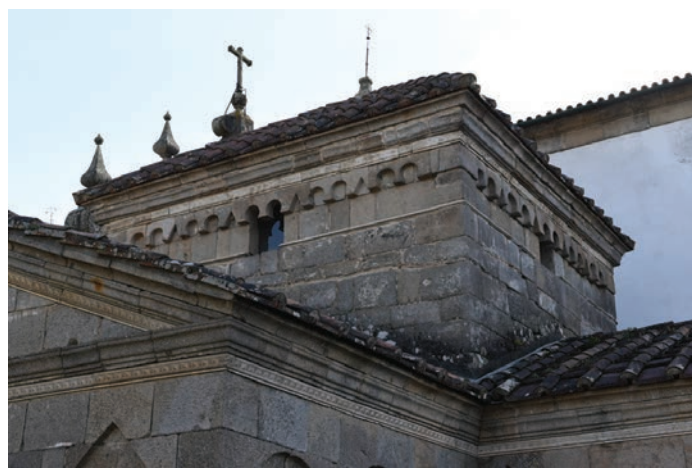
Fig. 9 – The exterior of the lantern-tower showing the frieze with alternating surpassed and mitre-shaped motives, and one of the small ajimez windows, truncated of the pillar
