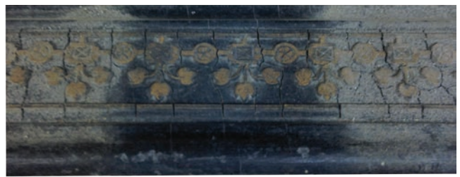
Sl. 24 Detalj - okvir u fazi čišćenja (foto: M. Petrović). Fig. 24 A detail of the the frame during the cleaning phase (photo by: M. Petrović).
