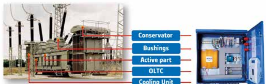
Figure 1. Example of transformer continuous on-line monitoring module to collect and analyse data from various sensors placed at strategic points of the transformer
