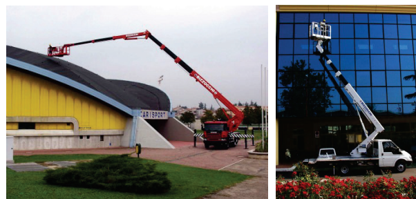
Figure 1 Use of platforms for maintenance and similar services
