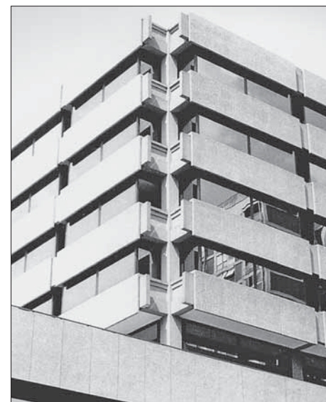
FIG. 7 ZAGREB, 'TEMPO' OFFICE BUILDING – SDK (SOCIAL ACCOUNTING AND AUDITING SERVICE), A. DRAGOMANOVIĆ, R. NIKŠIĆ, 1969-1981
