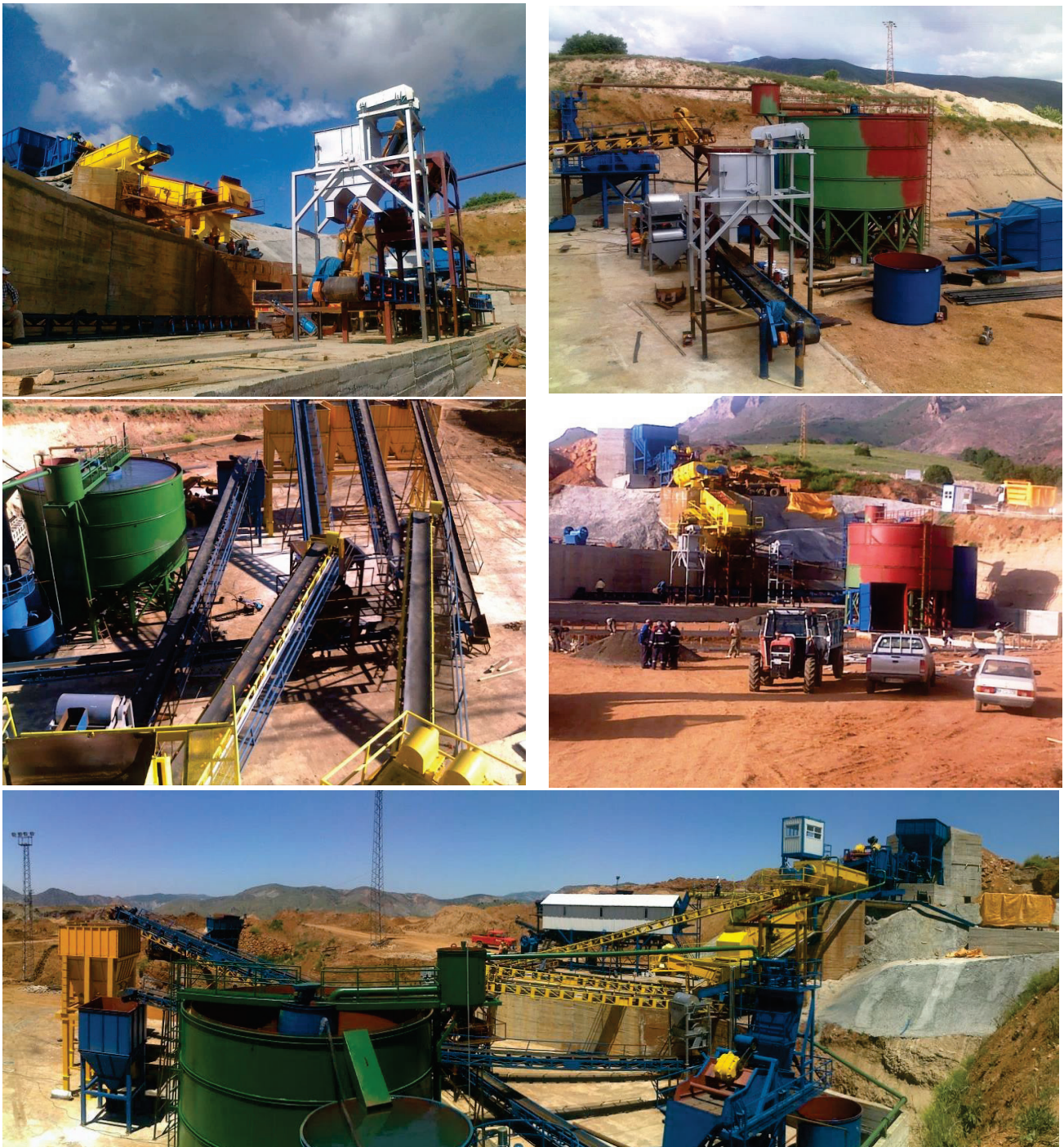
Figure 6 Building stage of the alternative flowsheet with 130 tph capacity in Divrigi-Sivas
