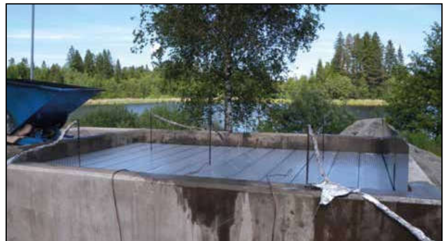
Figure 1: The transformer pit covered with the profile planks. Instrumentation consists of thermocouples and gas sampling probes. The tippable trailer on the left was used to contain the oil while being heated.
