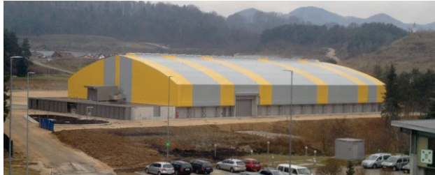
Figure 5 View of the biostabilization plant as a final stage of MBT
