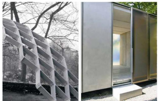
Fig. 1 TRC lattice structure and student café with TRC sandwich elements (source: BAUKO2, RWTH Aachen University)
