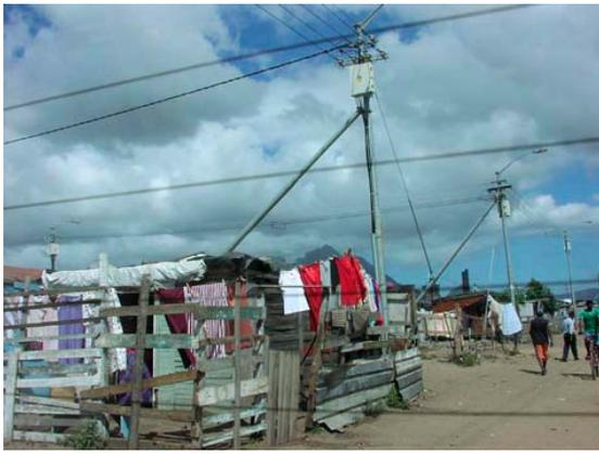
Fig. 2 Highly visible “maypole” type distribution system in Khayelitsha, Cape Town, South Africa makes electricity service drops less susceptible to theft [5]
