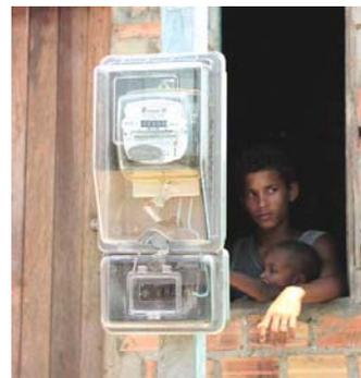
Fig. 1 Slum residents such as this mother with her child in Salvador, Bahia, Brazil now have a legal electricity service: the meter is a standardized "metallic kit" used to lower costs of slum electrification and to reduce stealing electricity [5]
