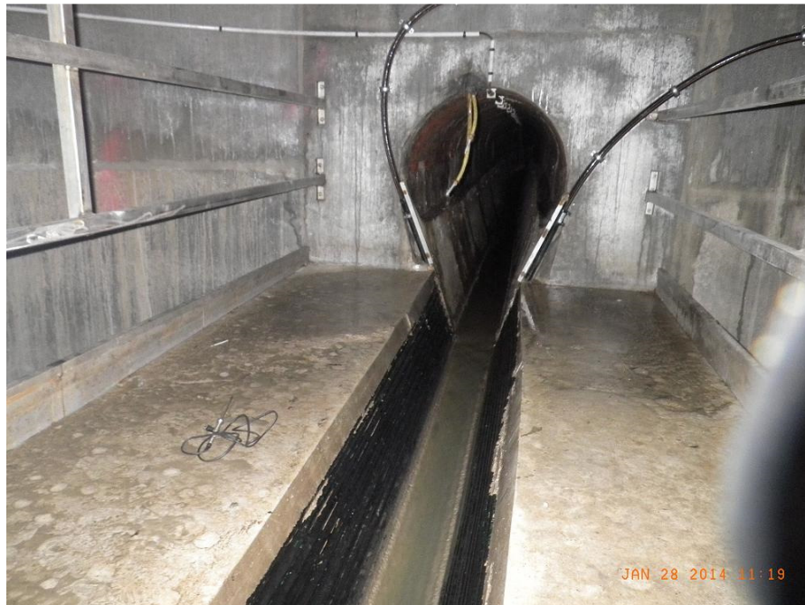
Figure 2. The heat exchanger at the MYRTES test facility
