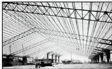
Figure 14 A frame system warehouse structure in Antwerpen [3]
