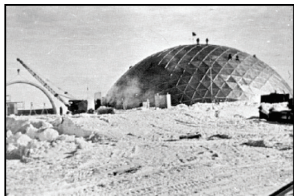
Figure 4 Aluminium dome research station in South Pole [3]
