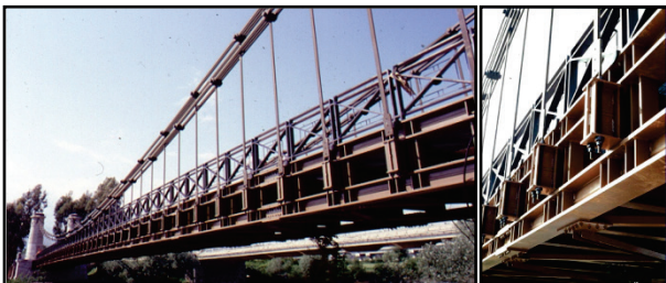
Figure 1 The Real Ferdinando bridge in Italy after re-construction – new aluminium deck [32]
