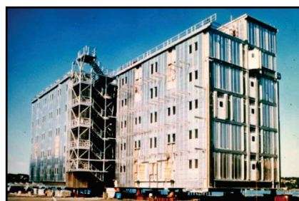
Figure 8 Accommodation module for an oil field before flout-out [17]
