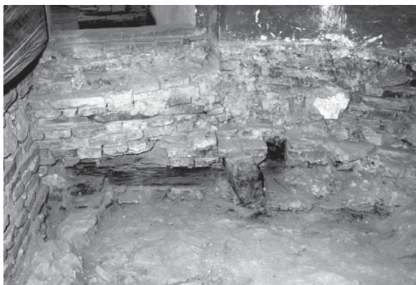
8. Dio prvotne nazidne grede kule C s ostatkom vezne grede i ležištem roga (snimila N. Vasić, 2010.) / Portion of the original wall plate of tower C with remains of joist and birdsmouth joint (photo N. Vasić, 2010)
