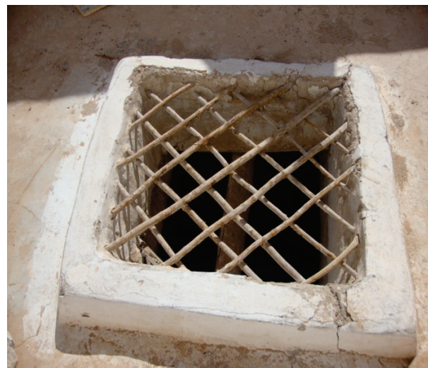
Figure 13 Opening at the roof
