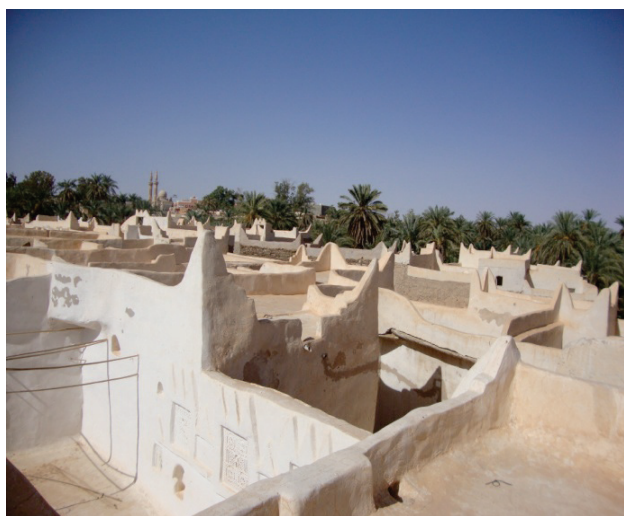
Figure 12 Roof for sitting and sleeping at night during summer
