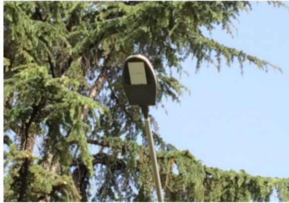
Figure 3. New LED luminaire
