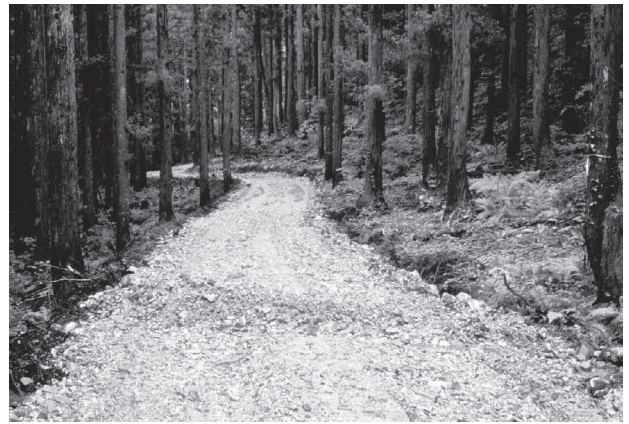
Fig. 13 Good sample of thick gravel on volcanic black soil
