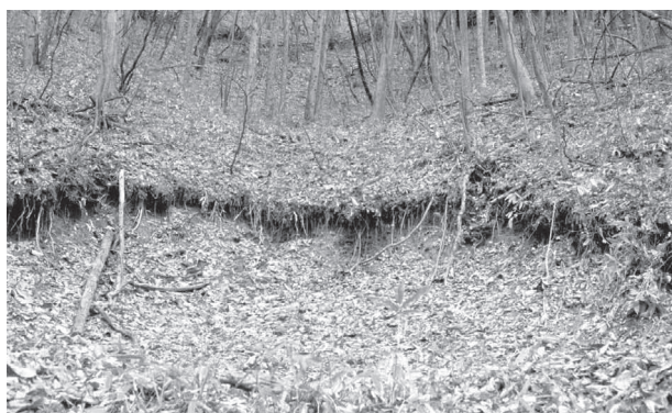
Fig. 19 Underwater is sometimes hidden under thick volcanic ash in such concaved slope and this can result in the collapse of the filling
