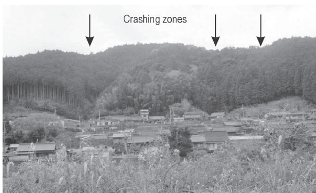
Fig. 17 Crashing zones can be found by irregular profile of the ridge line and a high tree at the ridge
