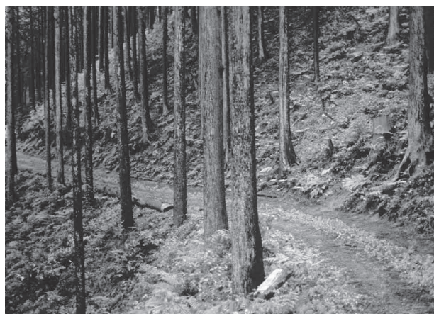
Fig. 10 Road by retaining wall with log structure at decomposed granite area
