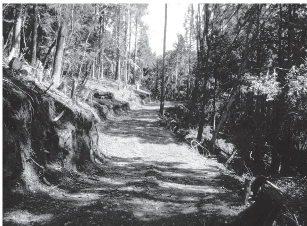
Fig. 23 Rolled grade whose sloping at lower sections is used for drainage
