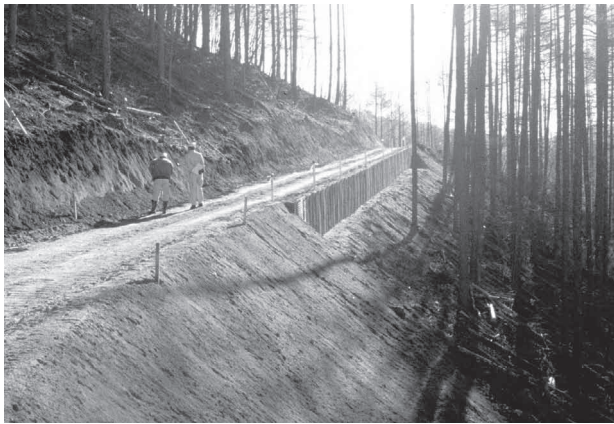
Fig. 11 Road construction with expanded mesh metal wall at decomposed granite area
