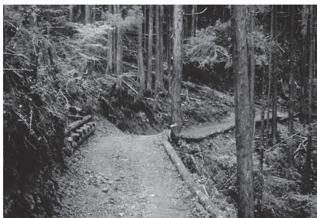
Fig. 7 Retaining wall with log structure both at cutting and fill slopes in Chichibu belt
