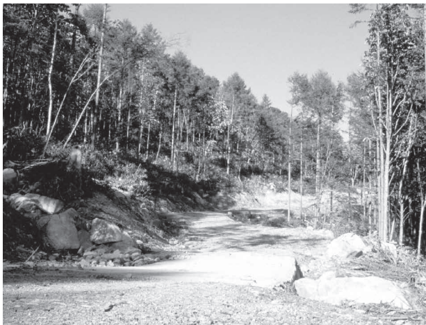
Fig. 20 Old alluvial fan area where old rivers are covered by sediment and/or deposit of debris flow and drainage facilities are required
