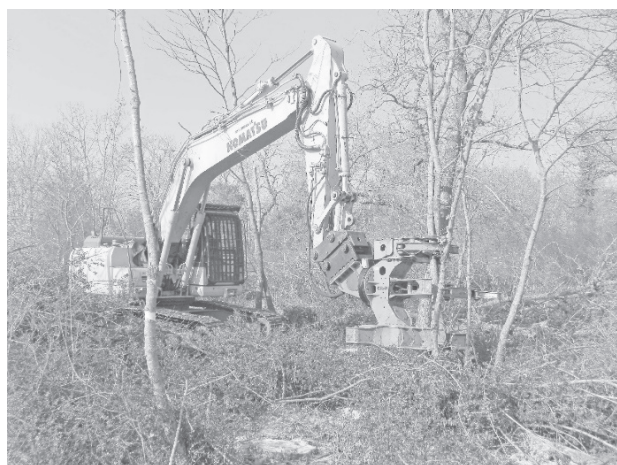
Fig. 3 Felling coppice with accumulating shears
