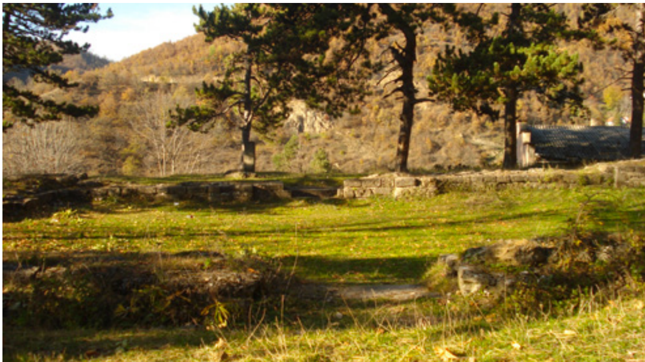
8. Stari Trg – Trepča, ostaci crkve sv. Petra, kraj 13. stoljeća, temelji, pogled s juga (foto: R. Ratkovčić) Stari Trg – Trepča, remnants of St Peter's church, late 13 th century, foundations, view from the south
