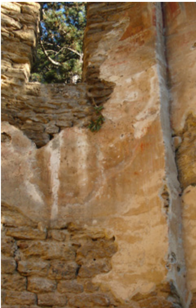
6. Stari Trg – Trepča, ostaci crkve sv. Petra, kraj 13. stoljeća, apsida s ostacima žbuke na kojoj su se nalazile zidne slike (foto: R. Ratkovčić) Stari Trg – Trepča, remnants of St Peter's church, late 13 th century, apse with the remnants of plaster where wall paintings were formerly located
