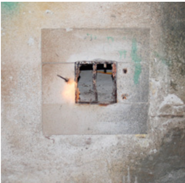
10. Odušak za zrak na barutani u tvrđavi sv. Nikole (foto: I. Glavaš) Air vent at the gunpowder magazine in St Nicholas' fort
