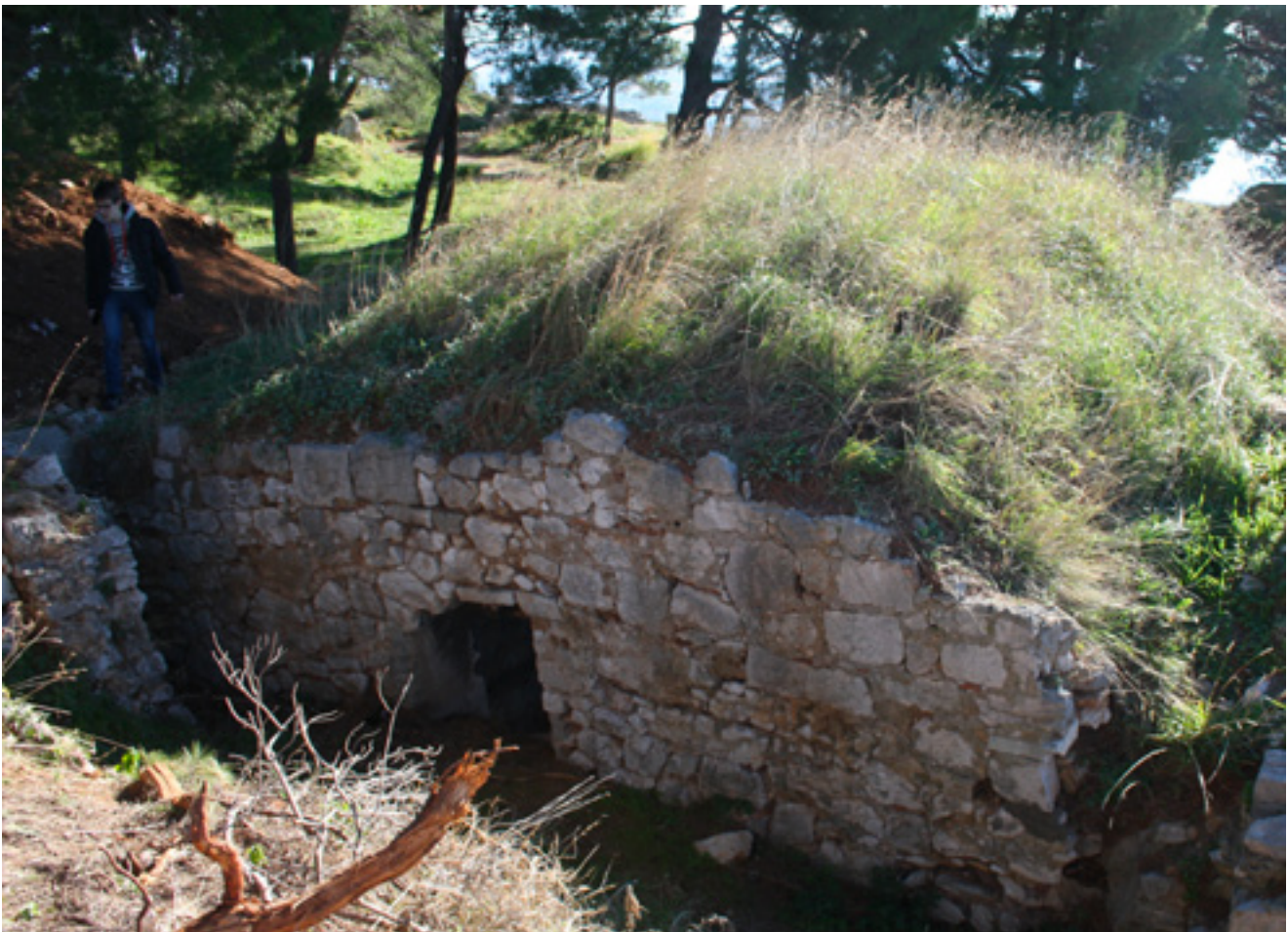
20. Pogled odozgo na krovšte barutane na tvrđavi sv. Ivana (foto: I. Glavaš) Bird's view on the roof of the gunpowder magazine in St John's fort
