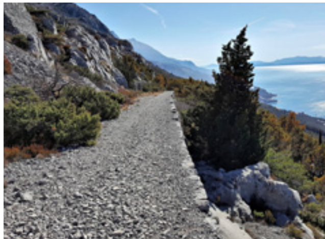
6. Uspon ceste ne prelazi 6%, gotovo prateći slojnice terena The road slant does not exceed 6%, almost following the terrain configuration
