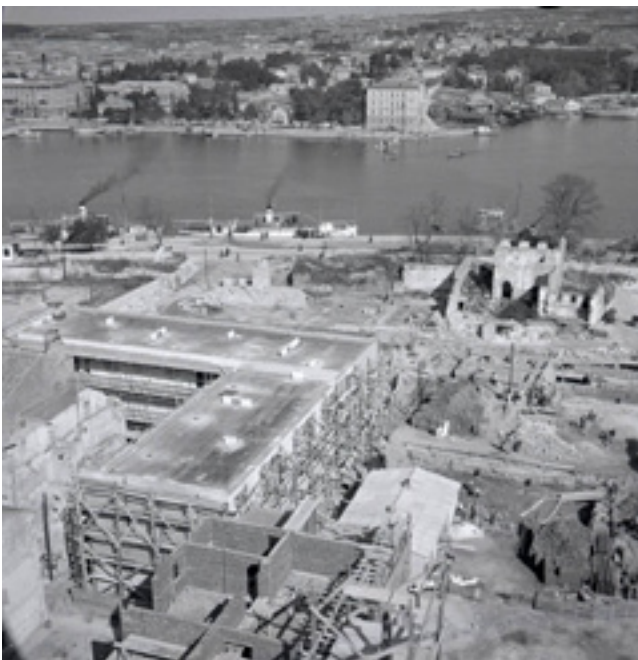
10. GU NMZ, fond Ante Brkan, pogled na Vitićev blok u gradnji Ante Brkan archive, view to Vitić's skyscraper in construction
