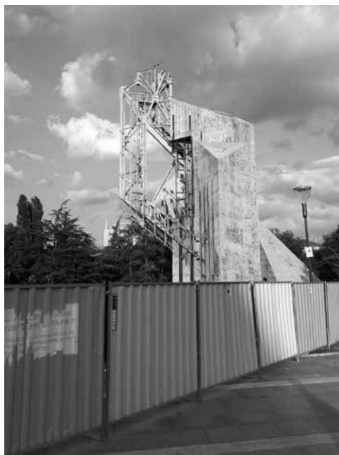
Figure 6: The Demolition, July 14 2017. Photo: Valery Gyurov. Source: Facebook
