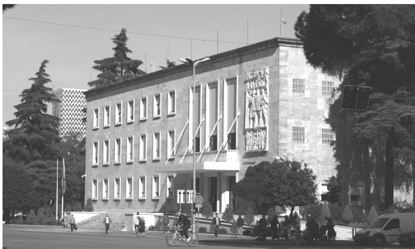
Figure 3: Prime Minister Building, Arch. Gherardio Bosio, 1942. Photo: R. Kodra
