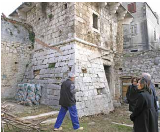
17 Spoj zidova dvorišta i Čorićevog tornja (foto: I. Glavaš) Juncture between courtyard walls and Čorić Tower (photo: I. Glavaš)
