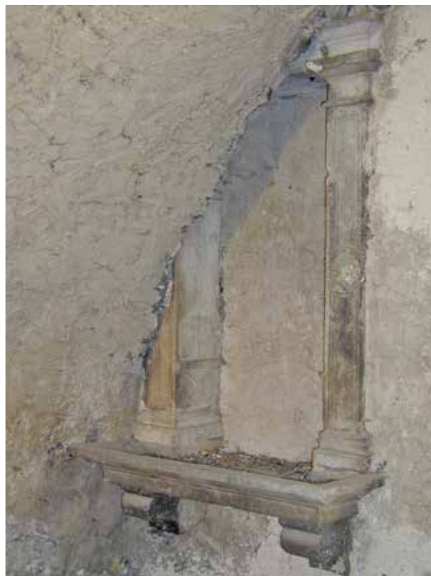
13 Renesansni kameni umivaonik na drugom katu Čorićevog tornja (foto: I. Šprljan) Renaissance stone washbasin on the second floor of the Čorić Tower (photo: I. Šprljan)
