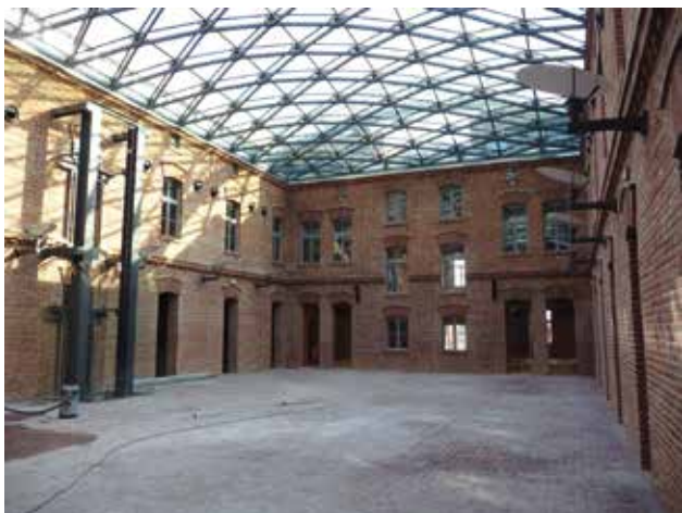
12 Home Army Museum building with inner glass-roofed courtyard (photo: W. Rymcza-Mazur, 2011).
