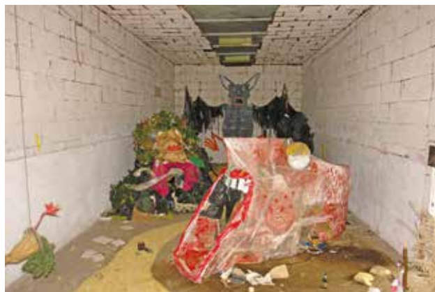
23 Unutrašnjost 1. kata nove hladionice (foto: K. Galović, 2017.) First-floor interior of the new cooling facility (photo: K. Galović, 2017)
