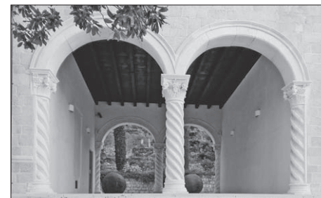
FIG. 18 RESTORED LOGGIA OF THE VILLA BONA-CABOGA ON BAHATOVINA (ART INSTALLATIONS BY THE PAINTER DUBRAVKA LOŠIĆ IN THE BACKGROUND)
