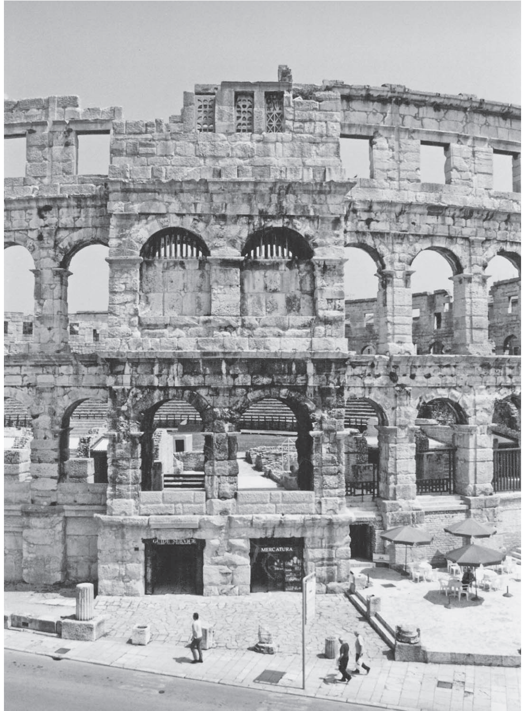
SL. 1. JUGOZAPADNI STUBIŠNI TORANJ 10-11-12 NAKON OBNOVE DIJELA SUTERENA I PRVOGA CIRKULARNOG HODNIKA FIG. 1 SOUTHWESTERN STAIRCASE TOWER 10-11-12, AFTER RECONSTRUCTION OF A PART OF THE SUB-GROUND LEVEL AND THE FIRST CIRCULAR PASSAGEWAY
