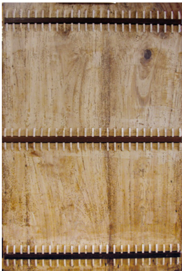
14. Novo poledinsko učvršćenje na slici sv. Martina (fototeka HRZ-a, snimila J. Baković, 2004.) New back reinforcement on the painting of St. Martin (Croatian Conservation Institute Photo Archive, photo by J. Baković, 2004)
