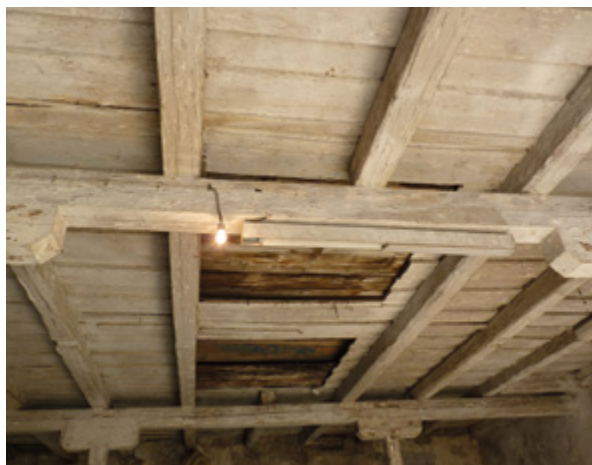
16. Drveni strop konjušnice s nekadašnjim otvorima za odražavanje (fototeka HRZ-a, snimila I. Pauk Sili) Wooden ceiling of the stables with former ventilation openings (Croatian Conservation Institute Photo Archive, photo by I. Pauk Sili)
