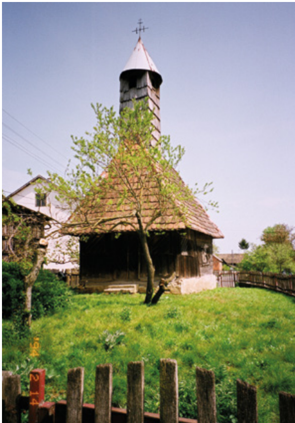
1. Zapadno pročelje kapele prije građevinske sanacije (fototeka HRZ-a, inv. br. I 130121, snimila J. Bartoniček, 1994.) West front of the chapel before the construction repair (Croatian Conservation Institute Photo Archive, inv. no. I 130121, photo by J. Bartoniček, 1994)
