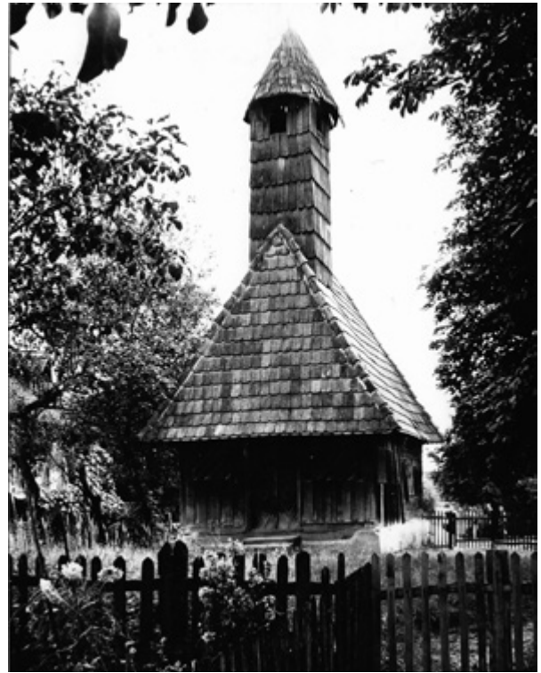
5. Pogled na kapelu nakon zamjene krovnog pokrova biber-crijepom, druga polovica 20. stoljeća (fototeka Instituta za povijest umjetnosti, inv. br. Stb.F-4, snimio I. Nikolić) View of the chapel after replacing the roof covering with beaver tail tiles, second half of 20th c. (Institute of Art History Photographic Collection, inv. no. Stb.F-4, photo by I. Nikolić)
