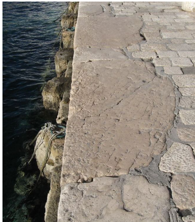
Fig. 7. Stone blocks built into the Hvar waterfront (Shore of St. Mark, Fabrika), built in 1554 (photo: M. Petrić)
