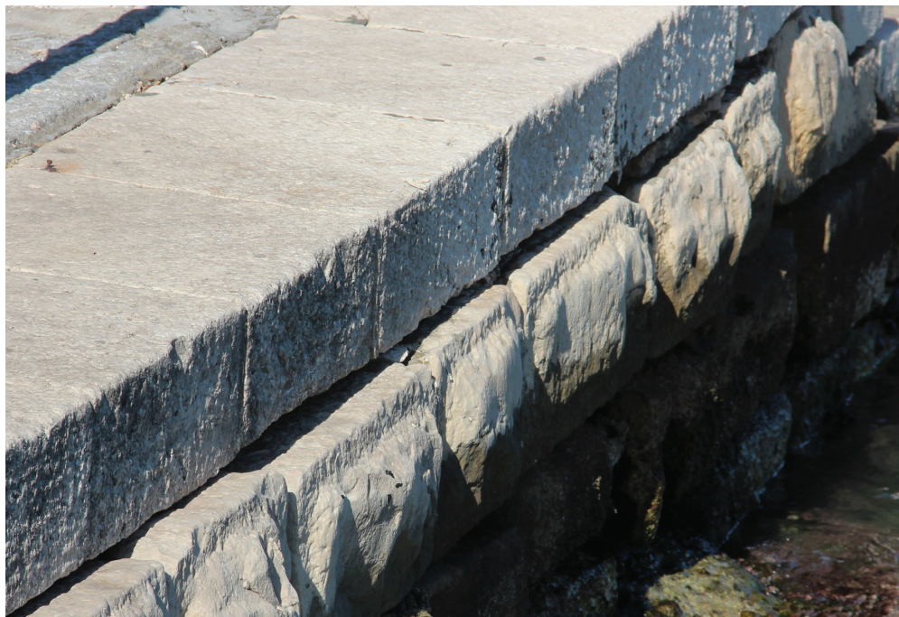
Sl. 4. Kameni blokovi ugrađeni u zidu obale na Žudiki kod mosta Trogir-Čiovo Fig. 4. Stone blocks built into the wall of the waterfront at Žudika near the Trogir-Čiovo bridge
