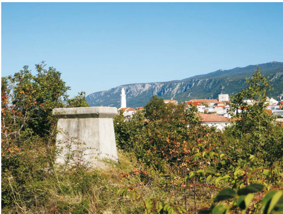
Fig. 5 Post of the Novi Vinodol astronomic point, today a 2nd-order trigonometric point. In the background is the tower of Sts. Philip and James' (sv. Filip i Jakov) Church in Novi Vinodolski. Photo by M. Lapaine, 2016 Slika 5. Stup astronomske točke Novi Vinodol – danas trigonometar 2. reda. U pozadini toranj župne crkve sv. Filipa i Jakova u Novom Vinodolskom. Snimio M. Lapaine, 2016.
