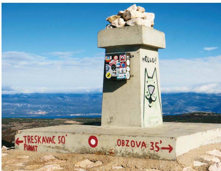
Fig. 7 Post at Veli Vrh point on the Island of Krk. The azimuth from the Novi Vinodol point was determined (1933–1936) toward this point. Photo by M. Lapaine, 2017
