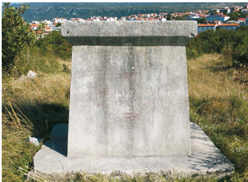
Fig. 6 Novi Vinodol astronomic point. The superscription on the post reads: Astronomic point, Military Geographic Institute, 1933. Photo by M. Lapaine, 2016
