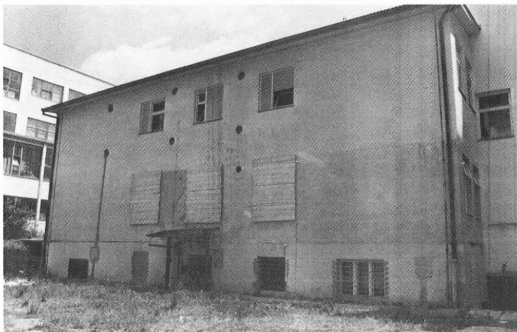
Slika 4. Daskama zakovani prozori bivše Intenzivne njege (snimio K. Đurak) FIGURE 4. The windows of the former Intensive care cheltered by boardings (Photo: K. Djurak)
