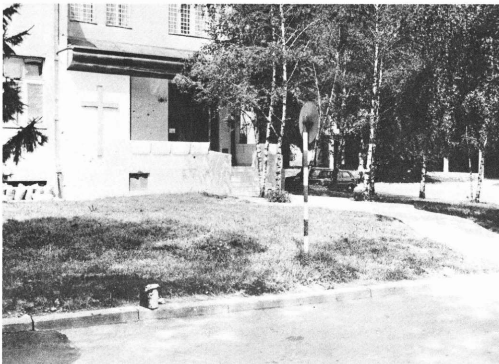
SLIKA 2. Zgrada odjela za zarazne bolesti poslije adaptacije FIGURE 2. The building of the Department of Infectious Diseases after the adaptation
